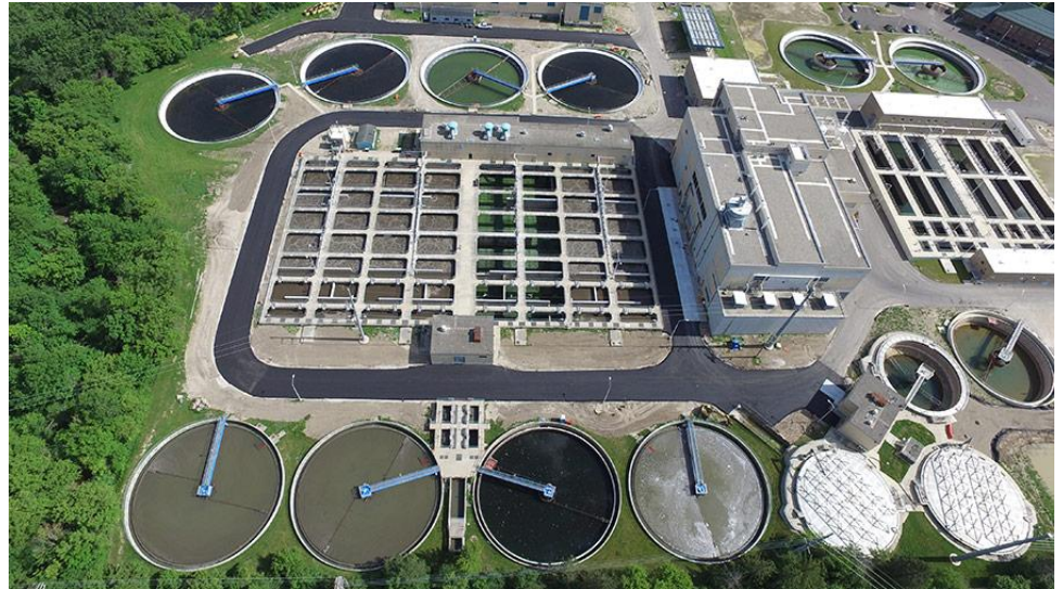
Figure 7: Aerial View of a Wastewater Treatment Facility [7]
