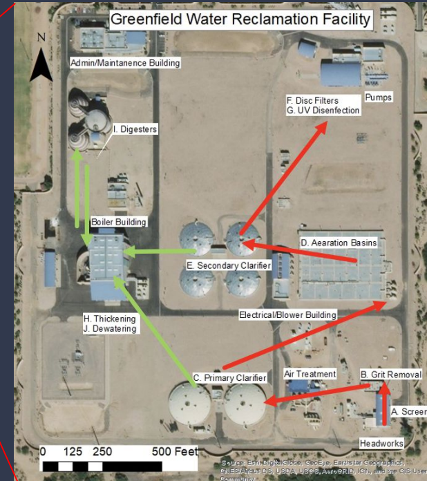
Figure 3: 2018 WEF Competition Wastewater Treatment Plant [3]
