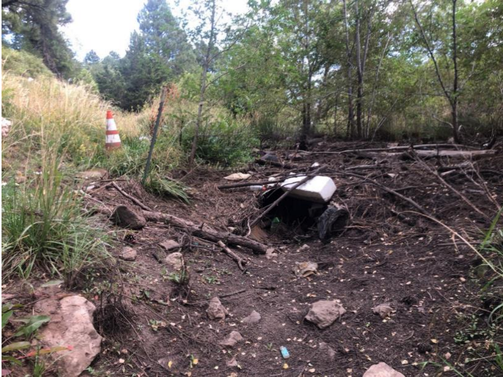
Figure 9-A: Upstream Culvert Undercrossing Bike Path
