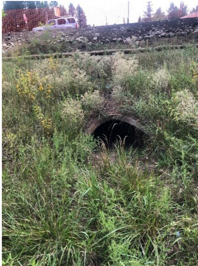
Figure 10-A: Culvert on Embankment along McConnell Drive
