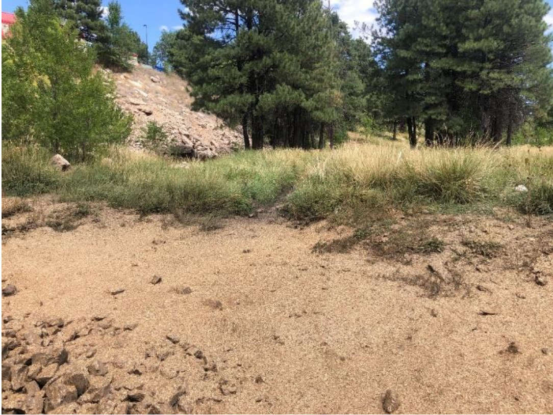
Figure 11-A: Downstream Channel Area by I-17 Overpass
