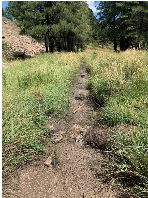
Figure 6-A: Channel of Wash looking Up-Stream
