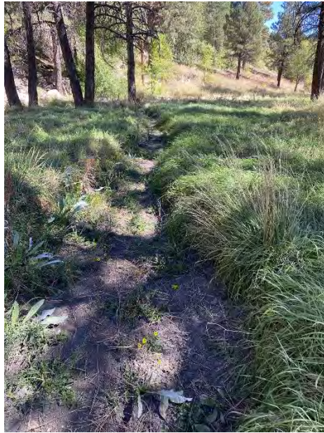
Figure 7: Station 1+40 Channel – Downstream
