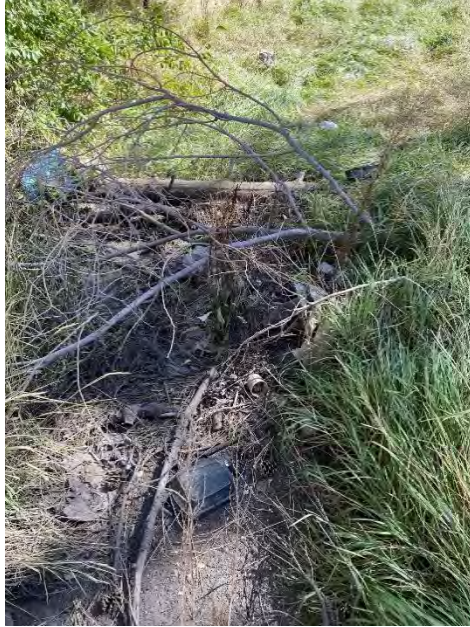
Figure 13: Station 2+10 Channel Obstruction
