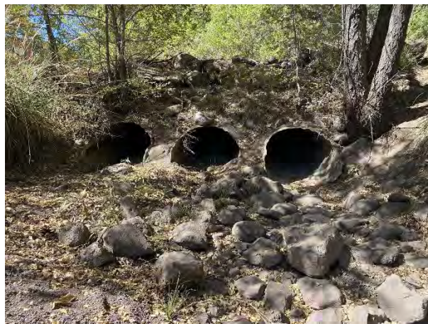
Figure 21: Culvert Outlets
