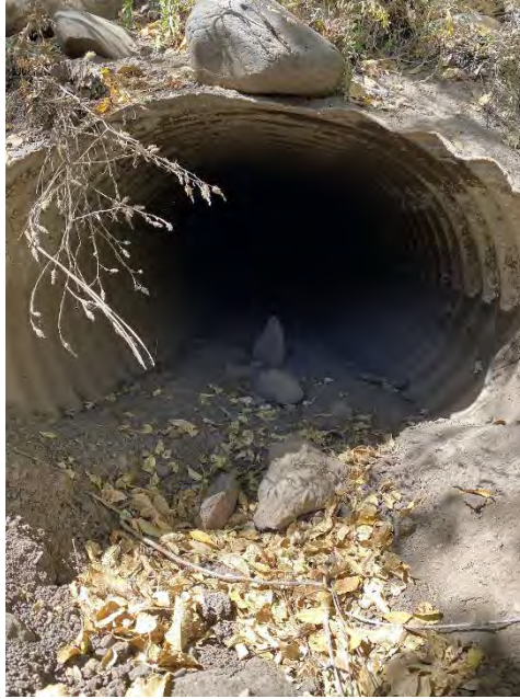
Figure 22: Left (South) Culvert Outlet
