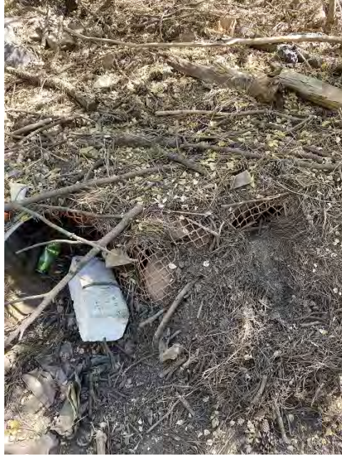
Figure 26: Culvert Inlet Conditions
