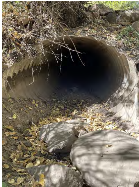
Figure 23: Center Culvert Outlet
