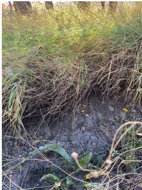
Figure 8: Station 1+40 Channel Embankment
