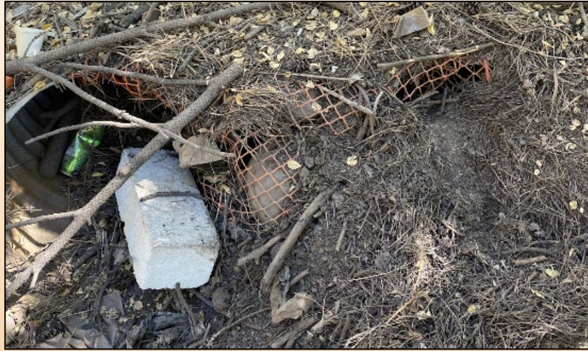
Figure 13: Culvert Inlet Conditions
