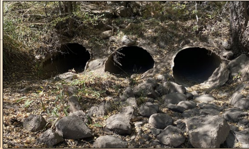
Figure 14: Culvert Outlet Conditions
