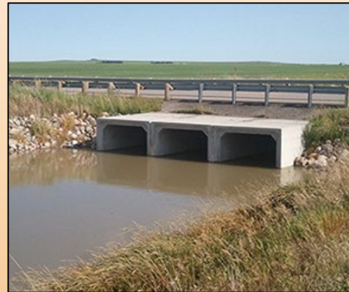
Figure 17: Triple Box Culvert
