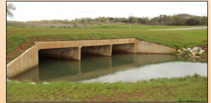
Figure 18: Triple box Culvert with Wingwalls
