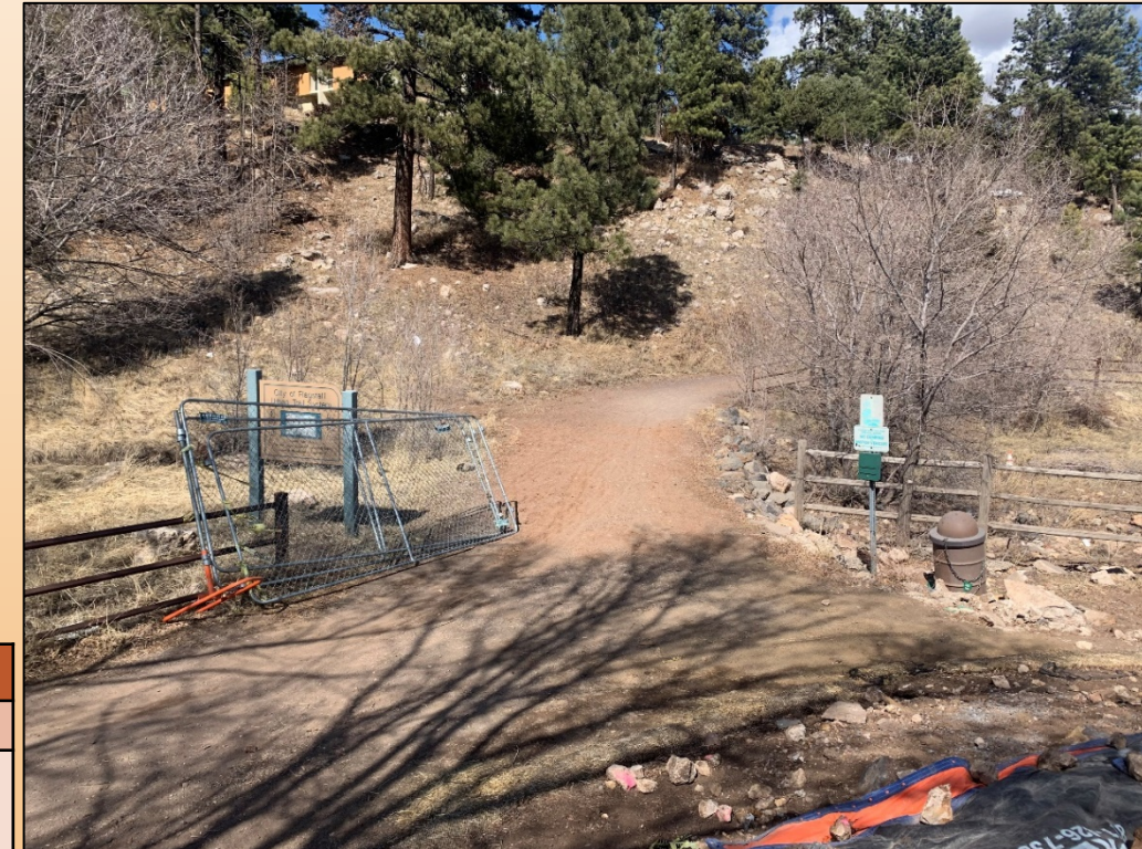
Figure 12: FUTS Crossing of Sinclair Wash
