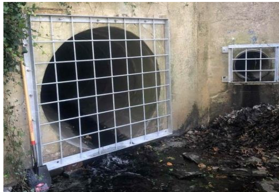
Figure 30: Culvert with Grate
