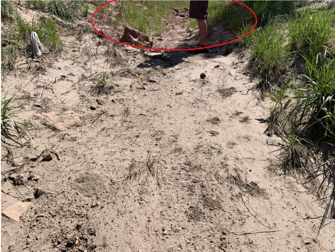
Figure 13: Site 3 looking upstream. Photo taken by Destiny Gourley.
