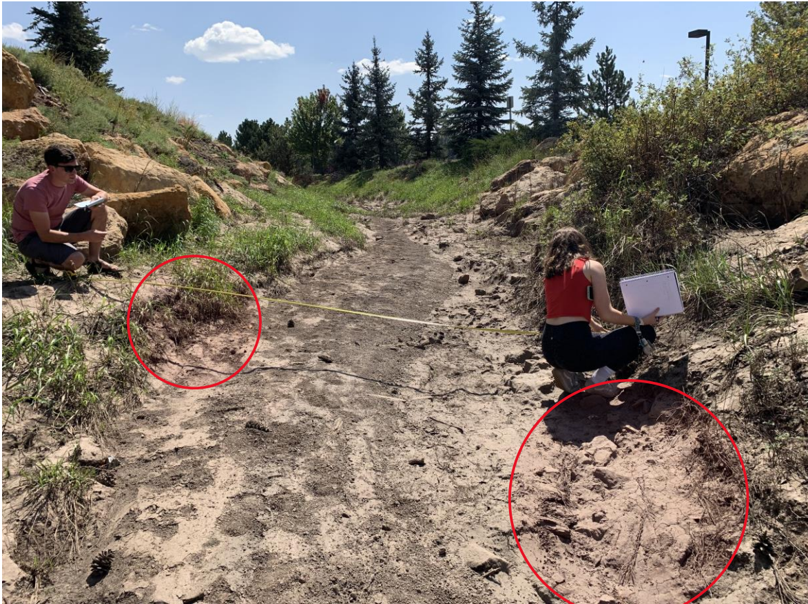
Figure 9: Site 1 looking upstream. Photo taken by Destiny Gourley.
