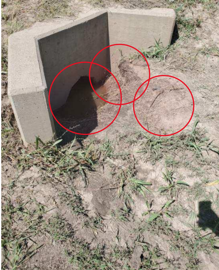
Figure 11: Influent culvert at site 2. Photo taken by Dan Segal.
