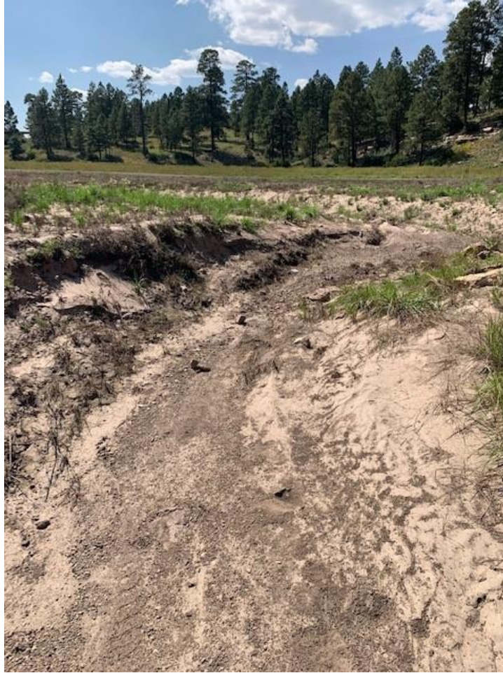
Photo Log 4: Rio de Flag channel station 54+77, looking upstream (south). This section of the channel shows silting, erosion, and signs of detention.
