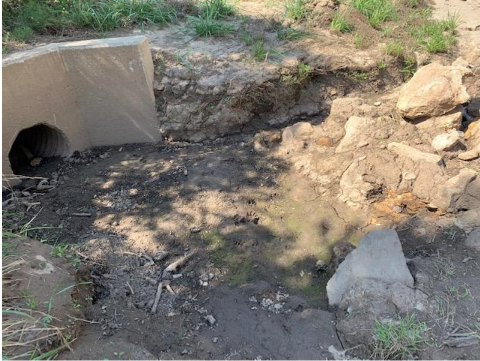
Photo Log 11: Rio de Flag channel station 79+35, looking downstream (north). This section is showing erosion, silting, and can be assumed detention would occur in the area if a flow was present.
