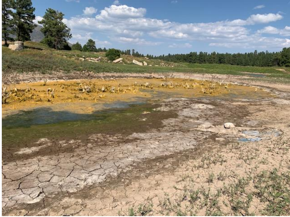
Photo Log 1: Rio de Flag channel station 23+42, looking downstream (north). This section shows retention and erosion.
