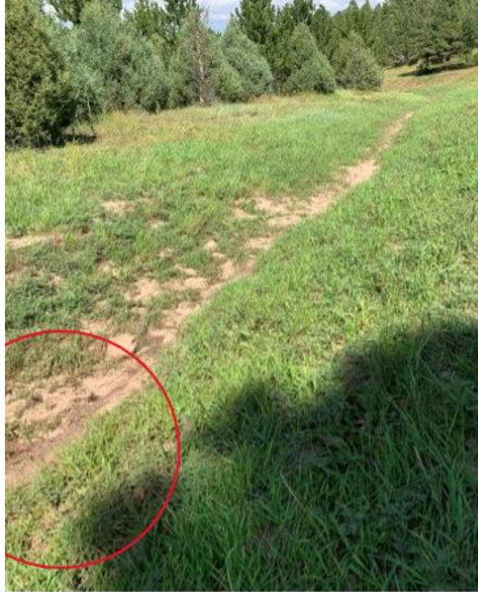
Figure 13: Image of Site 4, photo by Destiny Gourley
