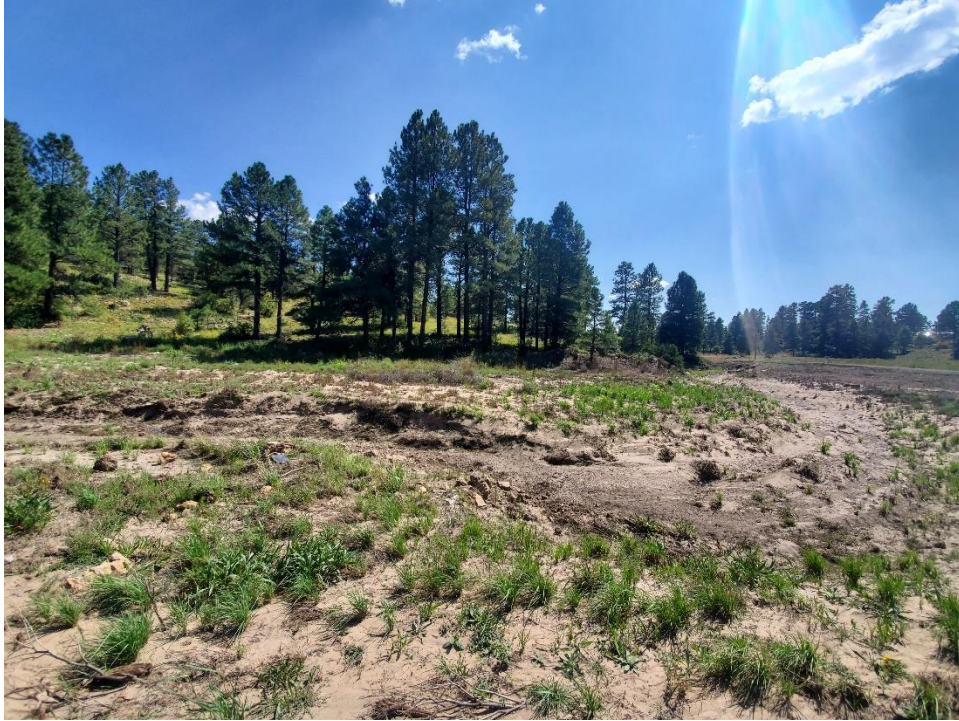
Photo Log 5: Rio de Flag channel station 55+14, looking upstream (south). This section shows silting and erosion.
