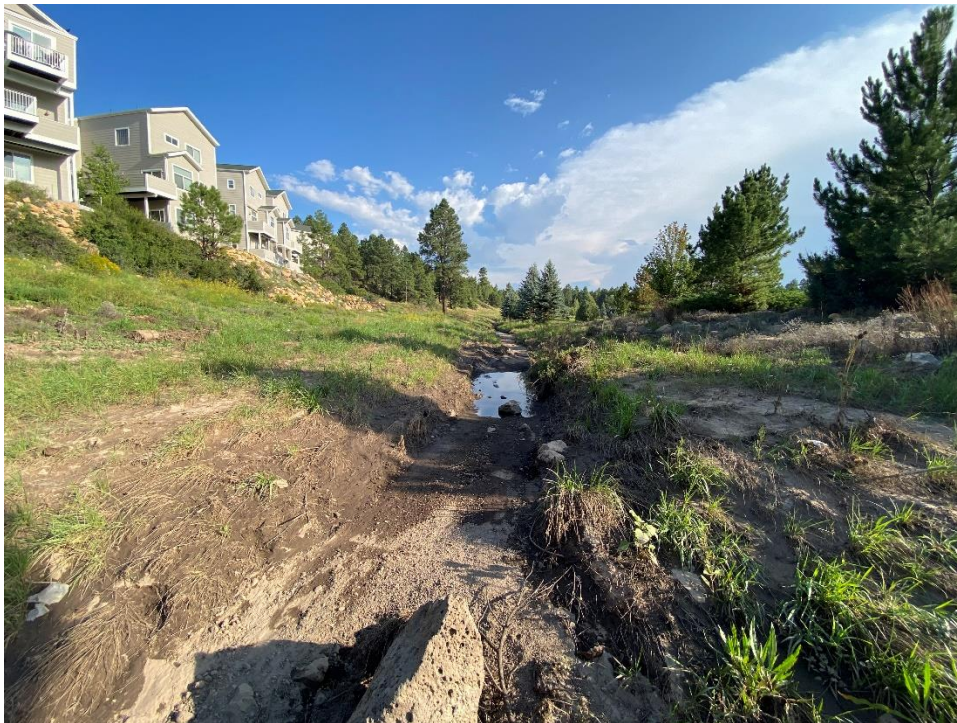
Photo Log 12: Rio de Flag channel station 80+78, looking upstream (south), this section of the channel is showing erosion, silting, and detention.
