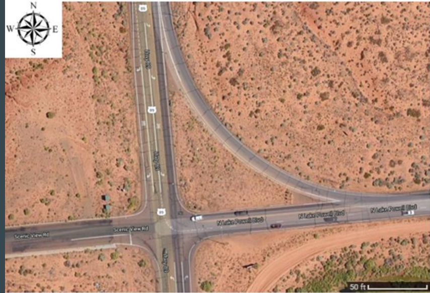
Figure 4 Aerial View of study intersection. Image Credit Google Maps [3]
