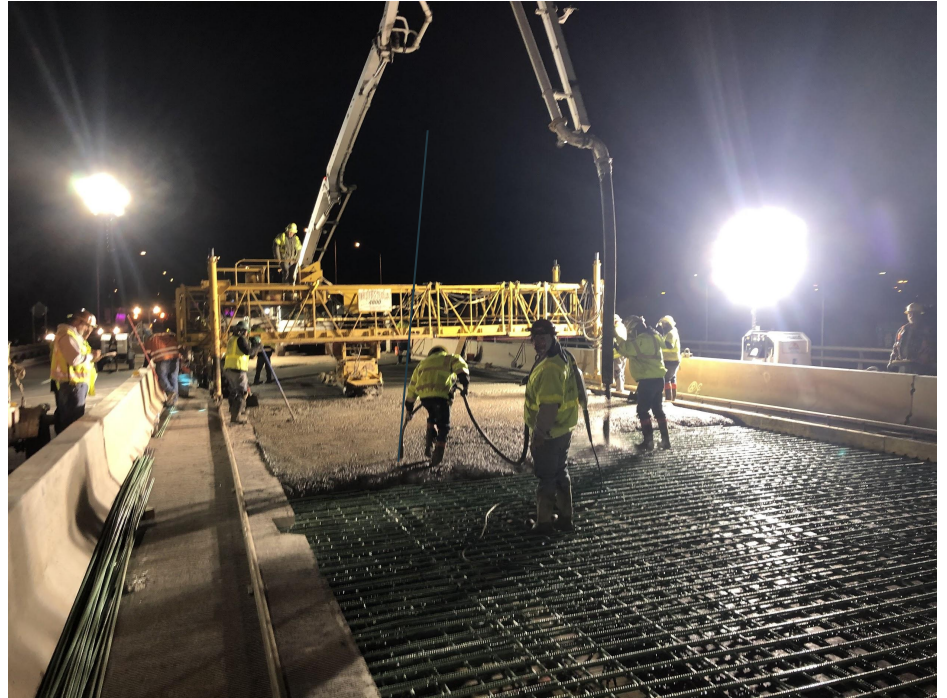
Figure 8: Roadway Construction (Flagstaff) [5]
