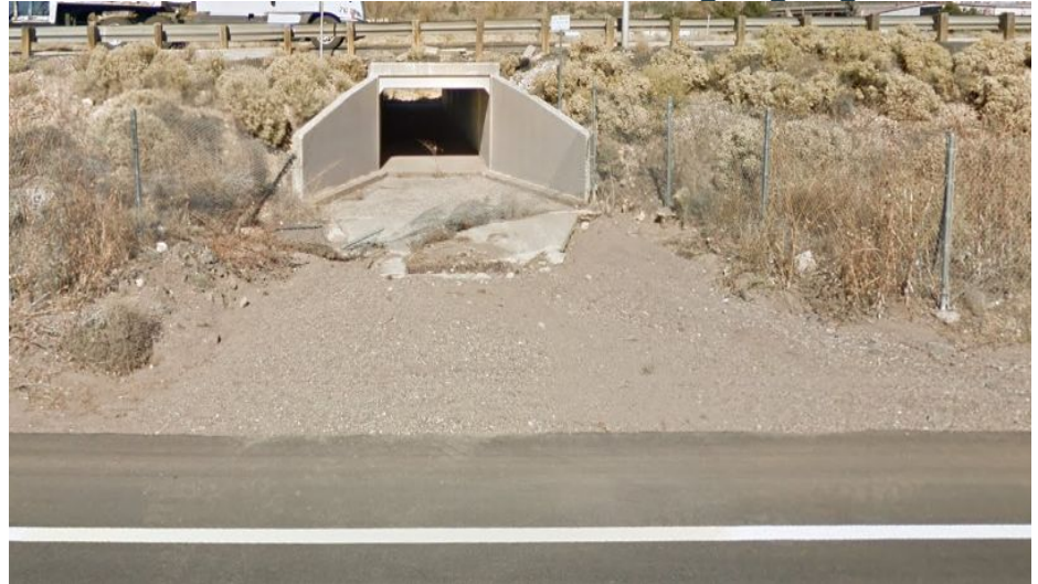
Figure 1: I-40E Existing Culvert [1]
