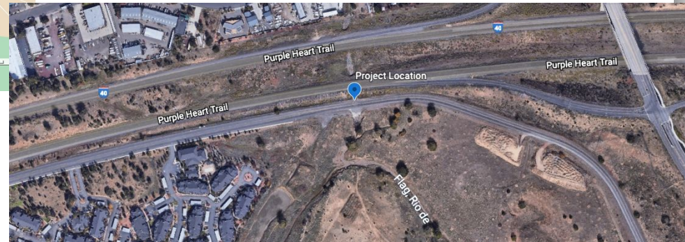
Figure 5: Aerial Image of Zoomed in Project location [1]
