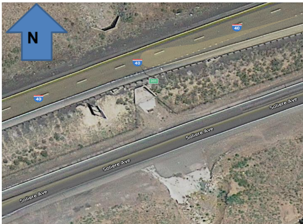
Figure 1.4: Project Location with I40 Culvert.
