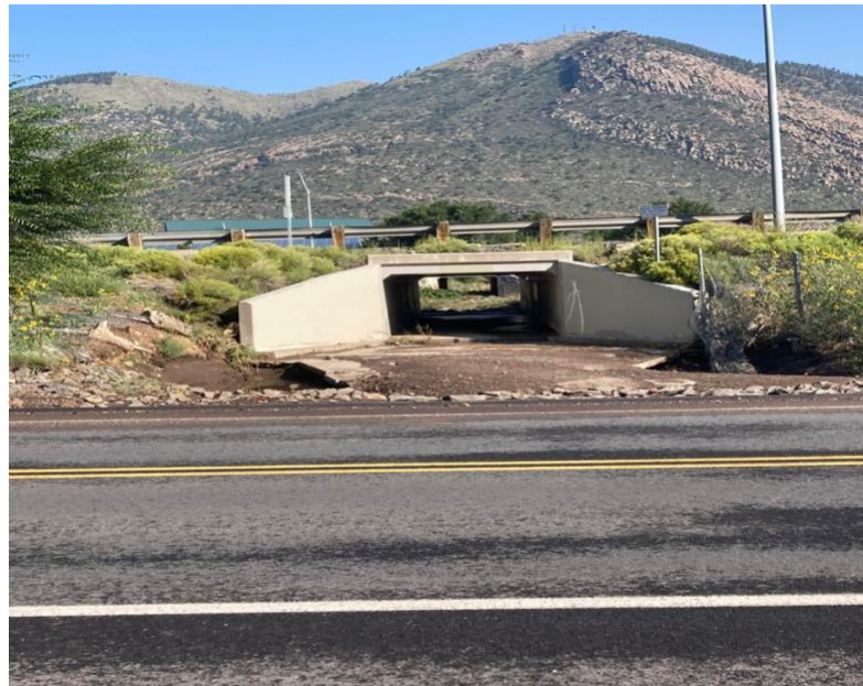
Figure 1.4: Existing I-40 Culvert
