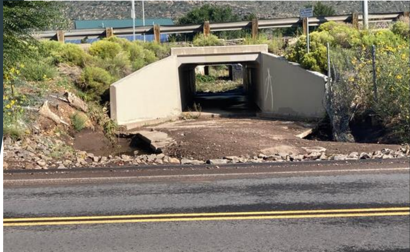
Figure 1: Soliere Ave running adjacent to I-40 Culvert
