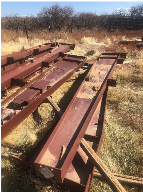
Figure 1: Center Rigid Supports on Site
