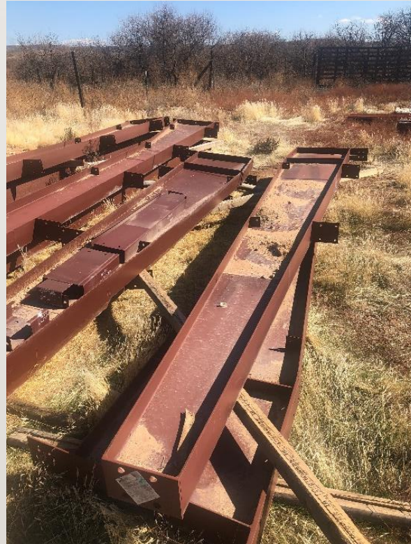
Figure 3: Center Rigid Supports on Site
