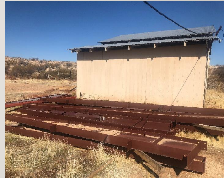
Figure 4: Center Rigid Supports Infront of Ex. Barn (34'x21')
