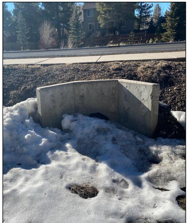
Figure 2. 2: Inlet Under Pulliam Dr
