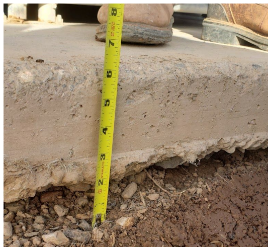
Figure 4: Measurement of the existing slab.
