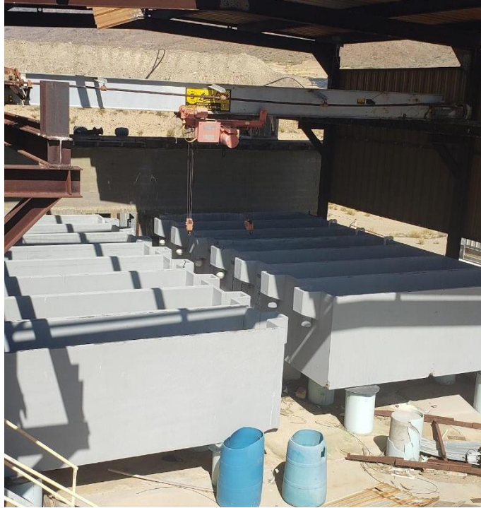
Figure 1.4: Abandoned Electrowinning Equipment (photo credit-Sydney Adamonis)
