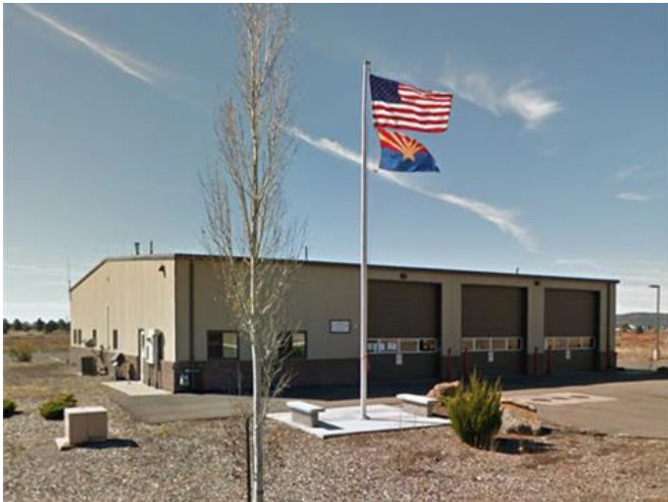
Figure 3: Street View of Existing Station
