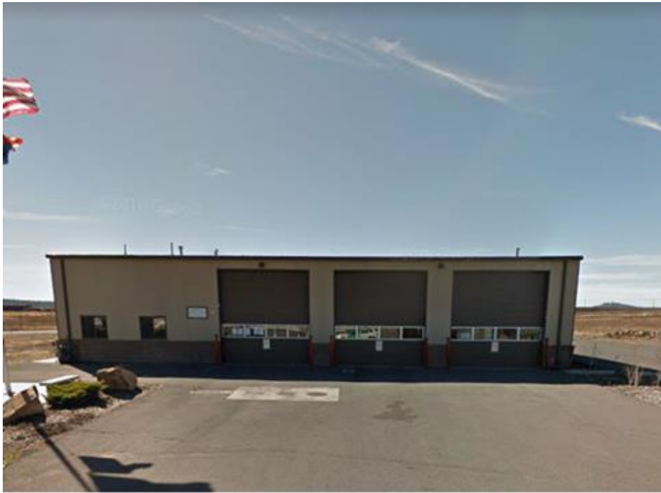
Figure 2: North Face of the Existing Station
