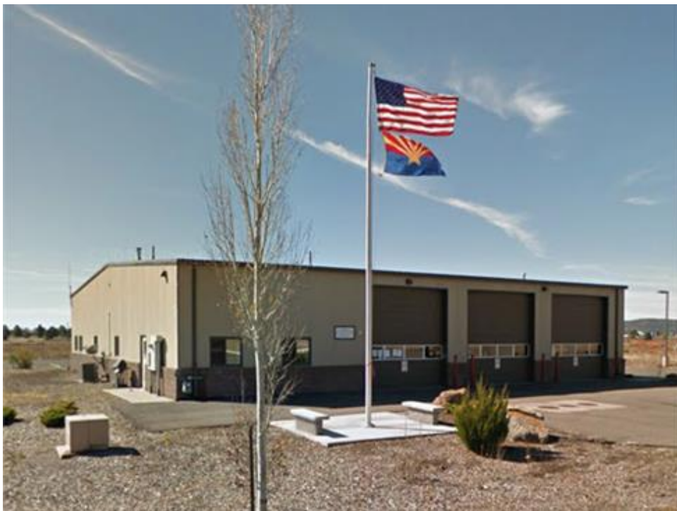
Figure 3: Street View of Existing Station
