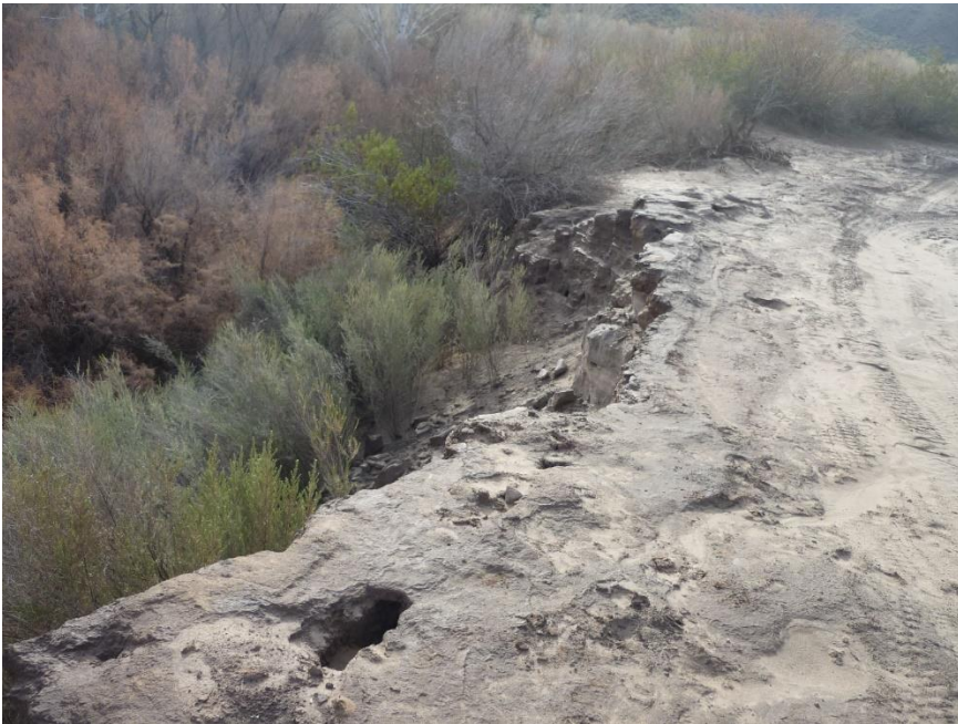
Figure C85. Signal Mill Slumping/Eroding Tailing Pile on the Eastern Side of the Site
