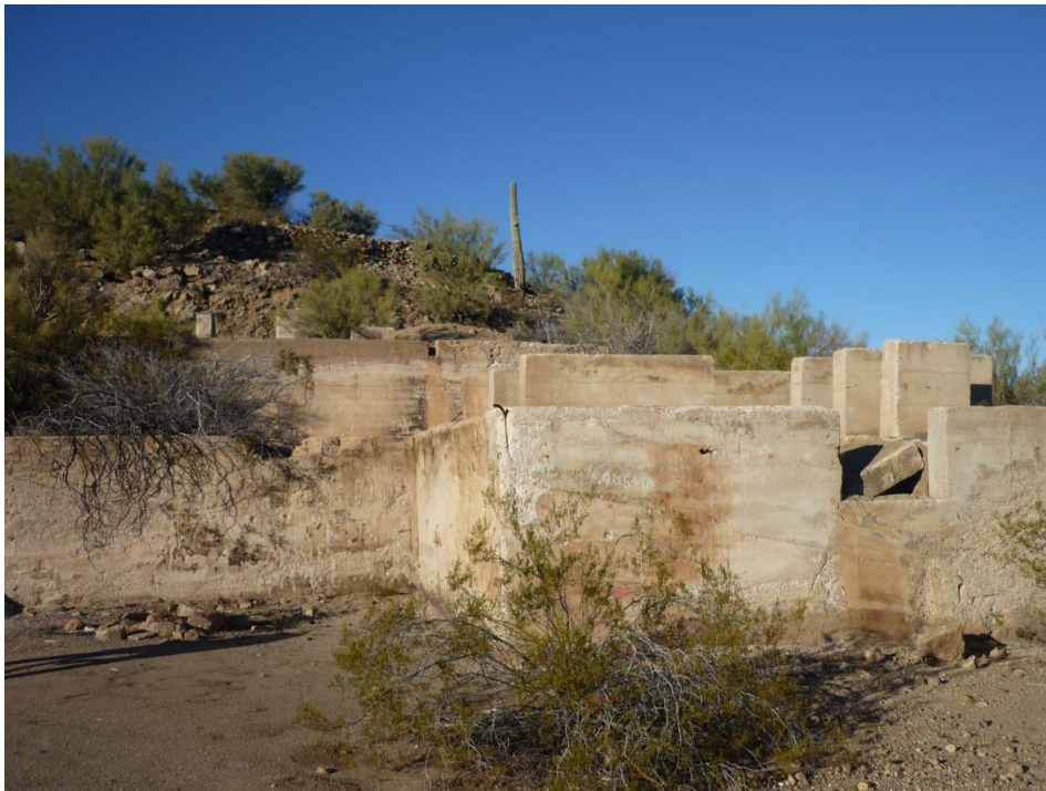
Figure C83. Signal Mill North Facing View of Concrete Structures on Site
