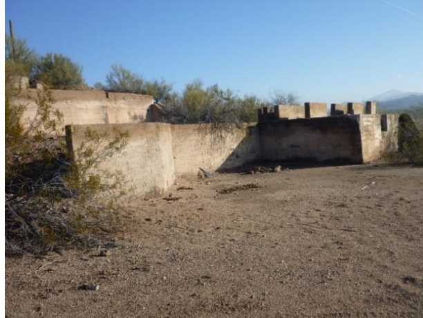
Figure 1.4 Abandoned Structure at Signal Mill
