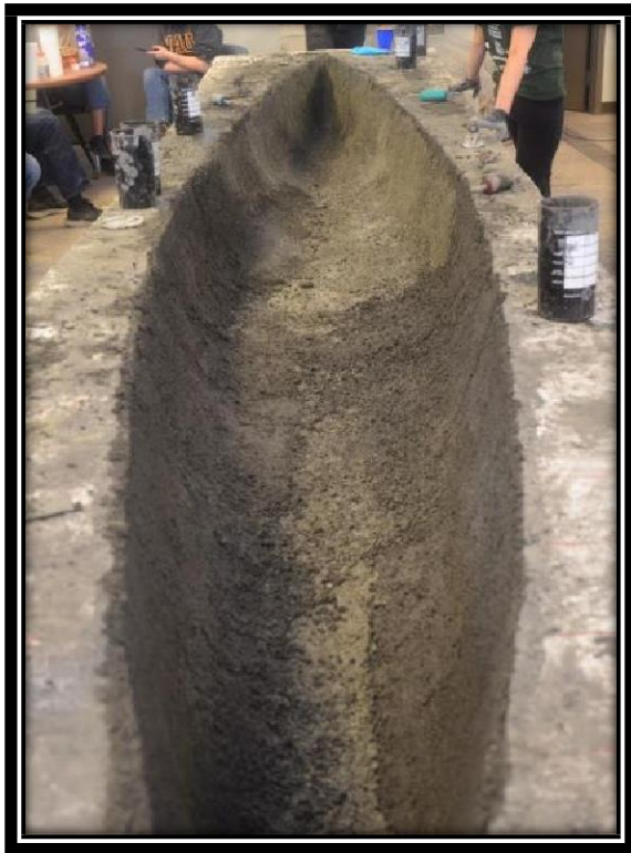
Figure 16: This picture shows the finished structural mix layer of concrete.
