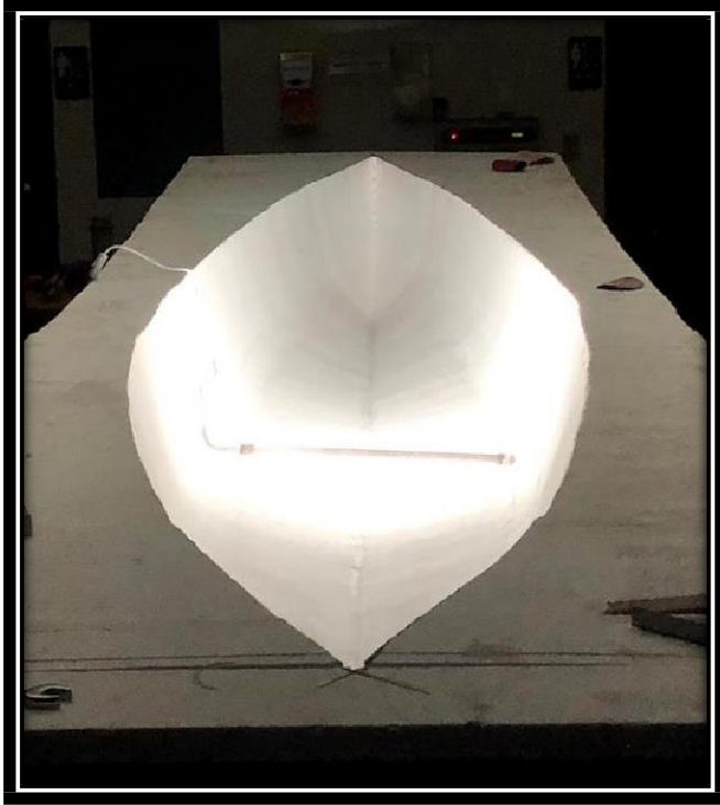
Figure 9: Shadow sanding was implemented by turning off all of the lights and using a single bright light to see any faults or uneven places of the foam. This helps make sure the canoe outline is smooth.
