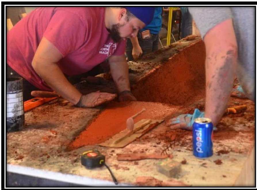
Figure 22: The end caps were covered with the red finishing concrete layer.
