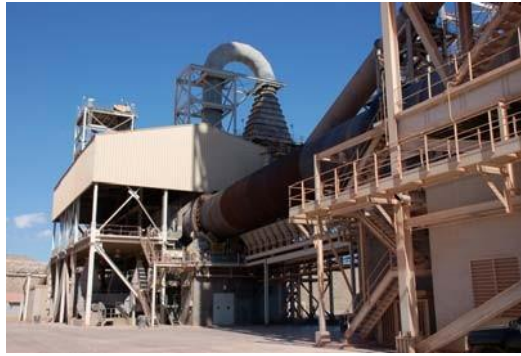
Cement Rotary Kiln, Clarkdale AZ
