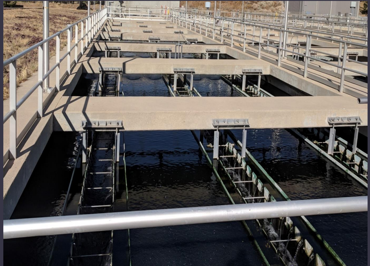
Figure 3: Wild Cat WWTP Secondary Clarifier Photo: Max Ward 5
