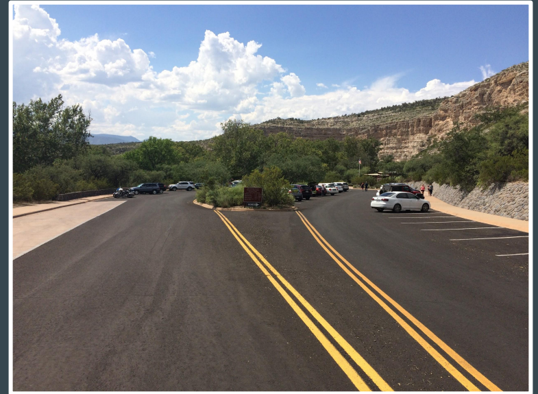
Figure 10: Looking West at the Existing Parking Lot Photo by: Andrew McLaughlin
