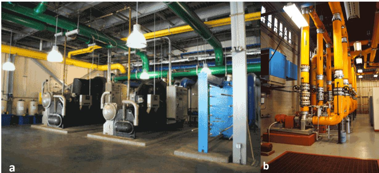
Figure 4: (a) The chillers inside the South Heating and Cooling Plant [8], (b) Part of the boiler system inside the South Heating and Cooling Plant [8]
