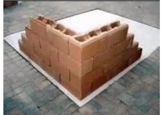
Figure 3: Dry Stacked Interlocking System [4]
