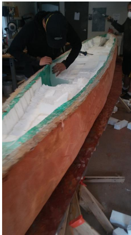
Photo 4. Removing Mold: A hot knife was used to cut through the styrofoam to properly removed pieces of the mold.
