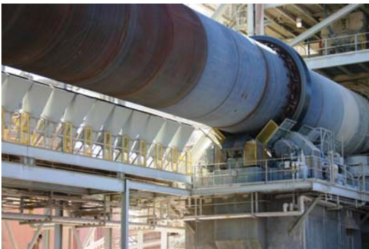
Cement Rotary Kiln, Clarkdale AZ
