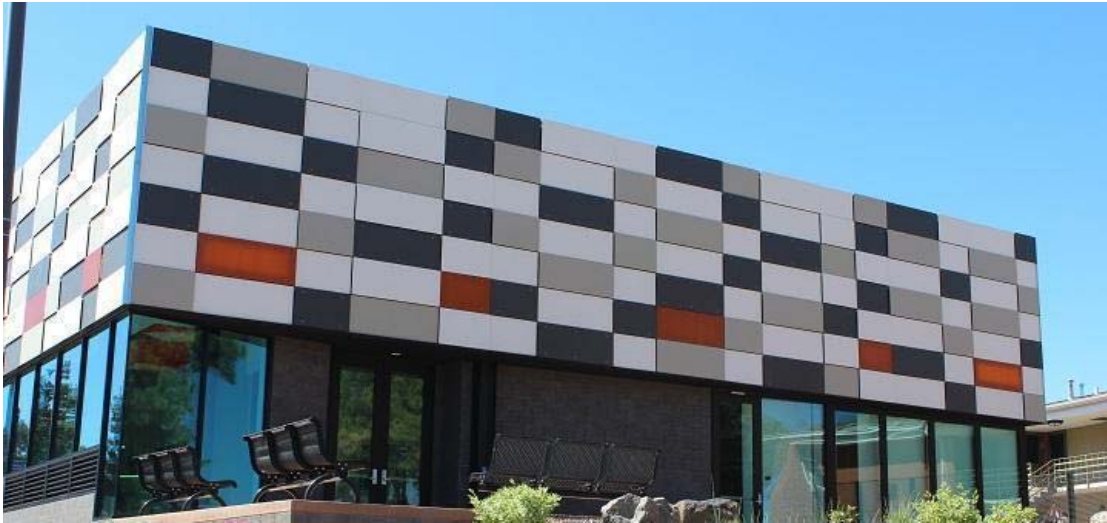
Figure 1.3 North elevation view of the existing building (looking south)
