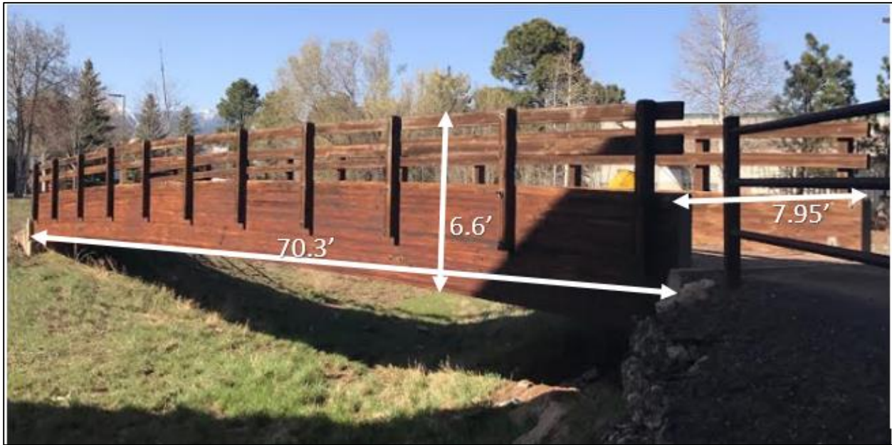
Figure 3: View of Existing Structure with Dimensions Annotated
