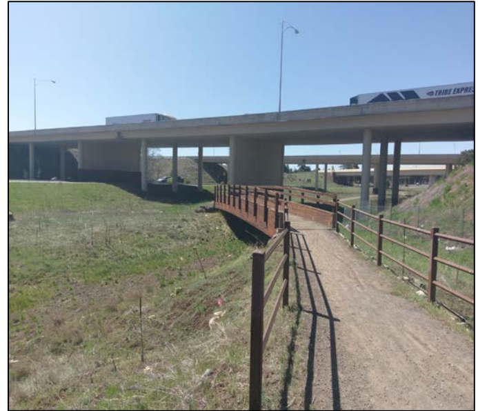
Existing Structure Facing South
