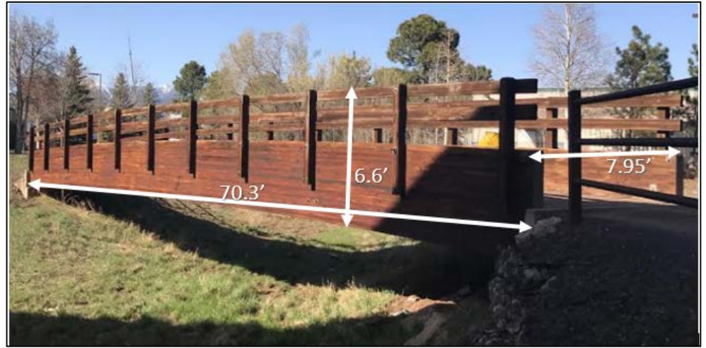
Dimensions of Existing Structure
