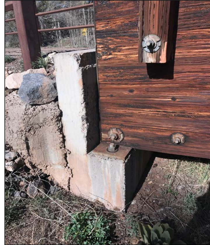
Pre-existing Footing at Project Site
