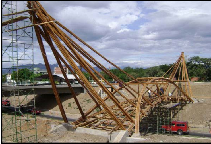
Bamboo Bridge being Assembled [1]
