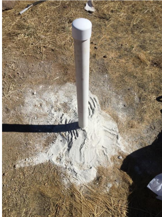
Figure 16: Packing the monitoring well with Bentonite
