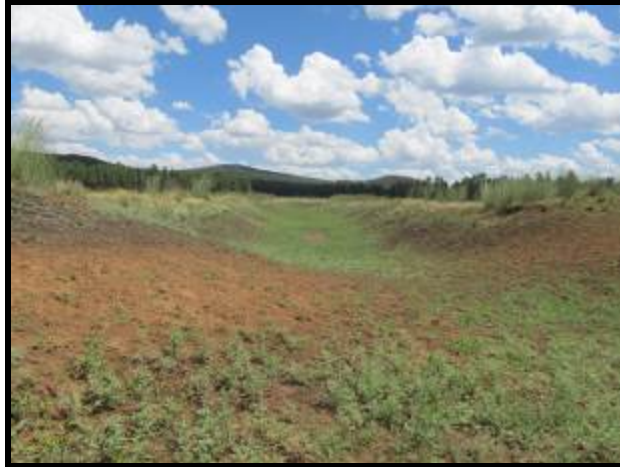
A ditch at Allan Lake 08/20/2013
