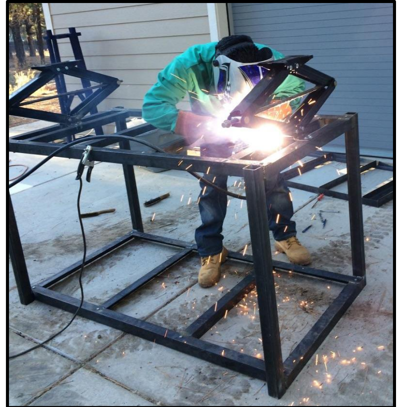
Figure 8: Welding of the Structure
