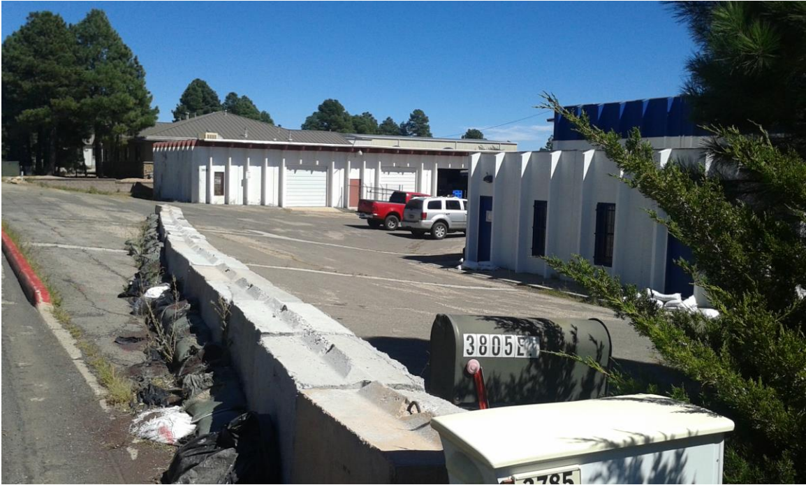
Figure 3-Barricades on Site (From Right of Building)
