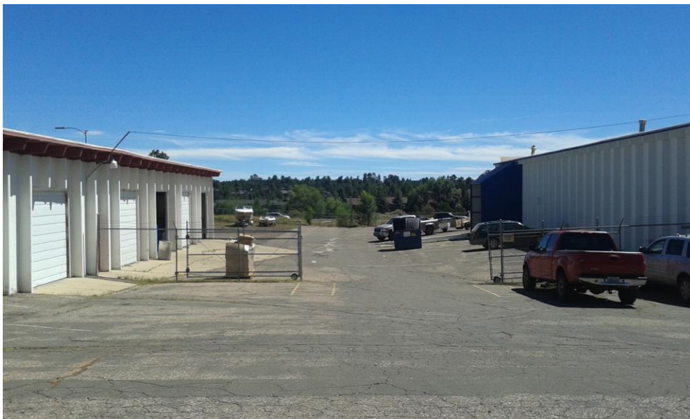
Figure 4-East Side of Food Bank Building
