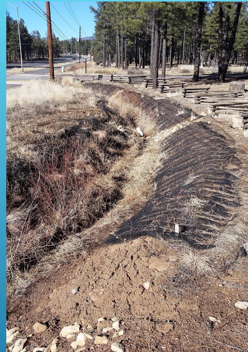
Turf Reinforcement Matting on Downstream End of Stream Looking North-West
