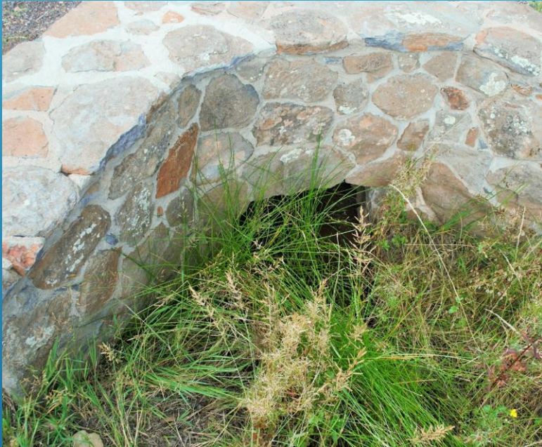
Above: Culvert 2 Inlet
