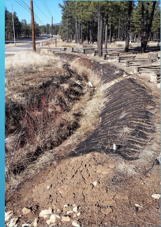
Above: Turf Reinforcement Netting
