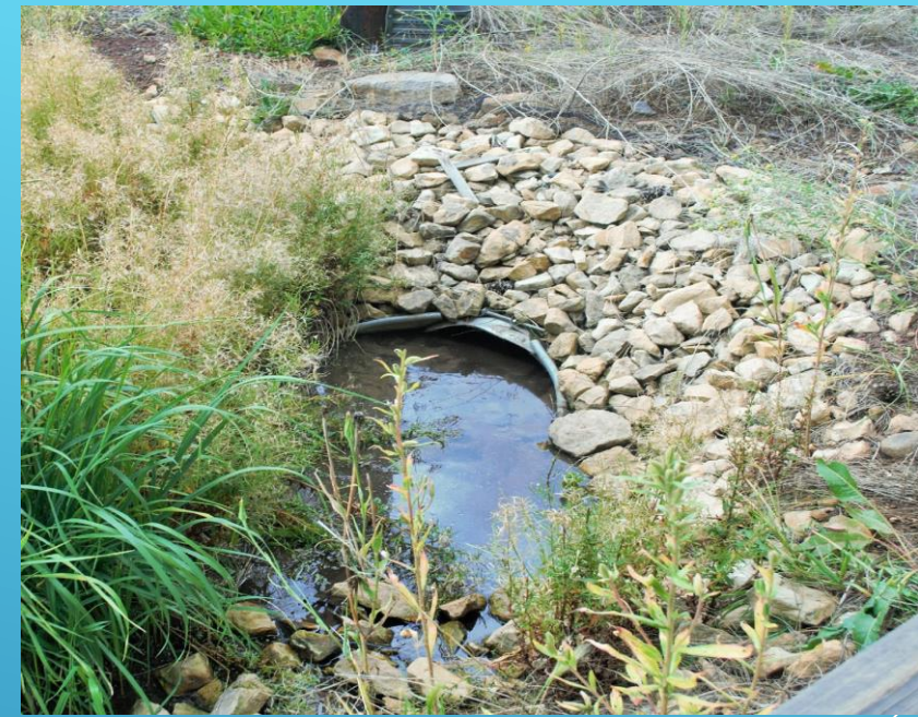
Above: Culvert 1 Outlet
