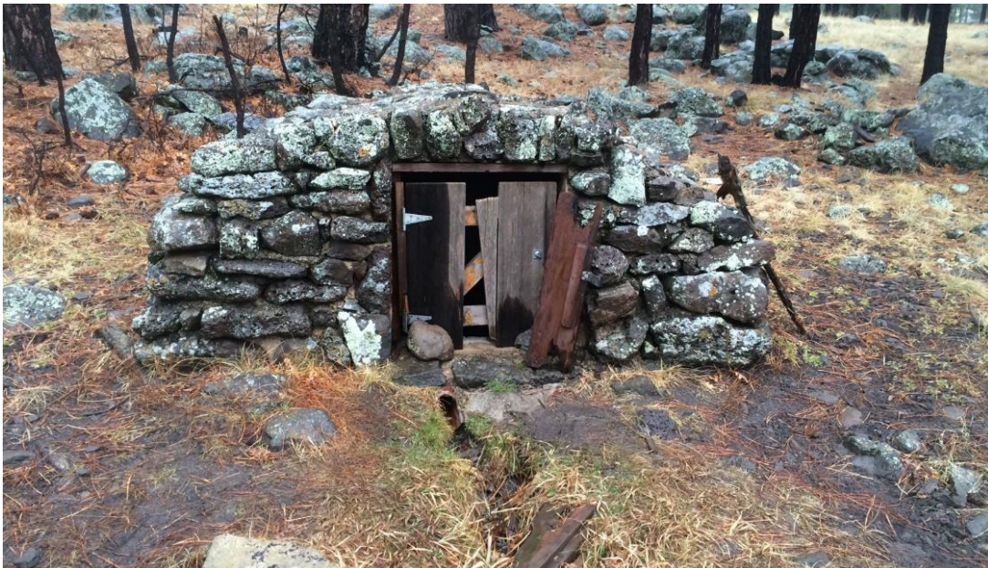
Figure 3) Coyote Spring Well House
