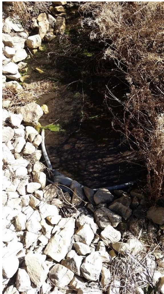
Figure 2) Culvert under Colton Ct.
