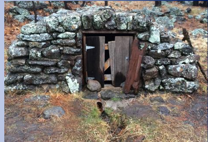
Coyote Spring Well House at Northern End of Project Site
