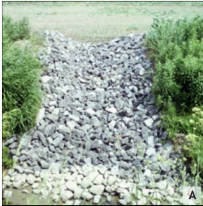
Figure 4. Rock Chute Spillway (Agriculture Canada)
