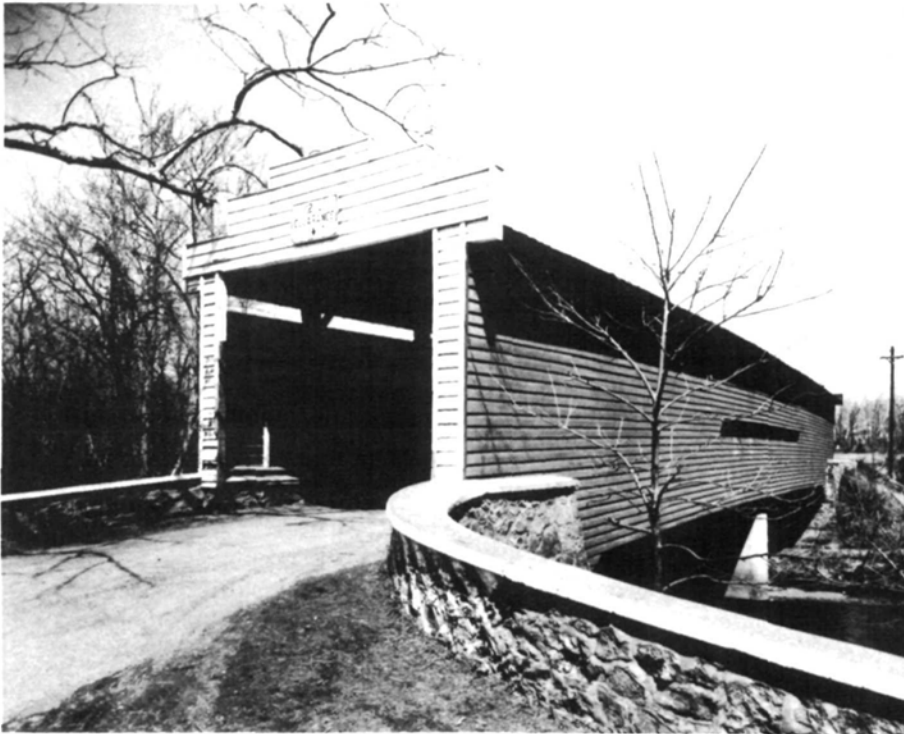
Hall's Bridge spanning French Creek, built about 1850 and 116 feet in length, is a surviving example of the Burr-truss design, which, invented in 1806, was a major advance in American bridge design. Over one hundred bridges of this type were built in Chester County, Pennsylvania, between 1812 and 1885. Hall's Bridge is one of the few remaining examples.
