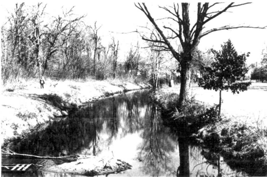
The Farmington Canal in Hartford and New Haven Counties, Connecticut, was constructed between 1828 and 1847. Along its 56 miles, the canal contains 28 locks, numerous bridges, culverts, and an aqueduct. (Historic Resources Consultants)
