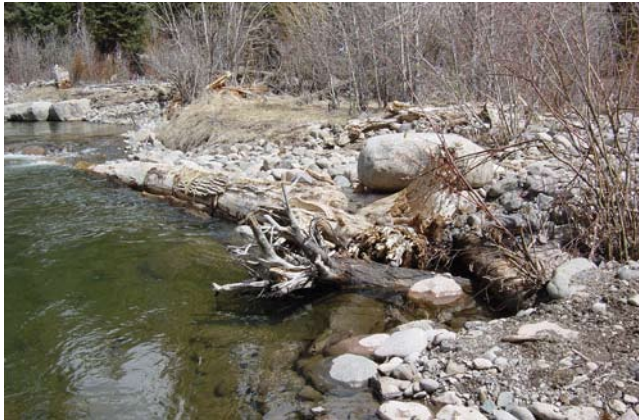
Figure 11-38 Rootwad/log vane/J-hook structure, East Fork Piedra River, CO
