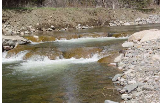
Figure 11-30 Cross vane/step-pool on the East Fork Piedra River, CO
