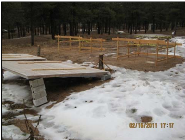
Figure 4: Roofs Waiting for Snow
