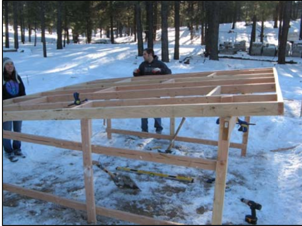
Figure 3: Construction Day January 8, 2011
